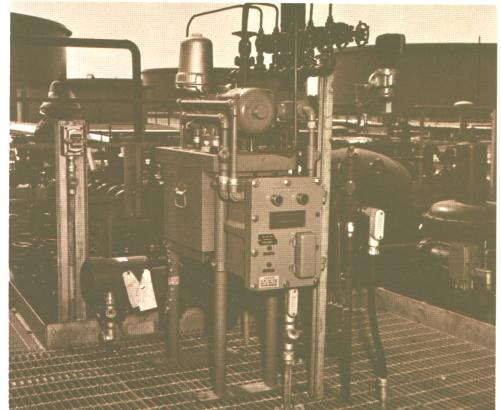
Demands for consistently high-quality products off the process stream have revealed critical shortcomings in conventional laboratory techniques of quality control. Laboratory procedures requiring analysis of samples drawn intermittently from the stream can occasion costly delays in correcting faulty output. The need for full-time monitoring of stream specification has given rise to the development of automatic, continuously operating process-stream analyzers.
